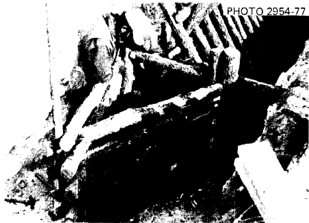
Fig. 11.4. The lower part of the vertical triangular entry is pressed horizontally against two pairs of vertical posts. Each pair is wired together. The two pairs are held apart by two horizontal spacer poles toenailed in place to frame the rectangular opening between the horizontal and vertical parts of the entry. The pairs of vertical posts are pressed against two horizontal poles (the uppermost is shown) that in turn press against both the outermost two poles of the horizontal part of the entry and the earth in two slots dug in the sidewalls of the excavation.
